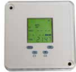
Seven-day timer for switching between melting temperature and lowered temperature
