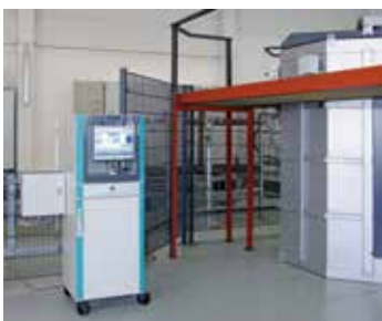
PC interface for central operation
